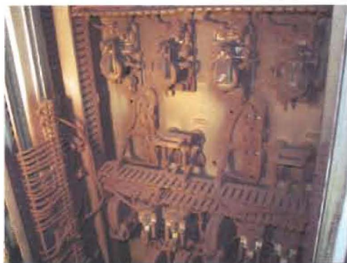
▲ BEFORE: Oily, mill dust, sticky accumulations cause outages and TIME to correct – when you can find the problem
